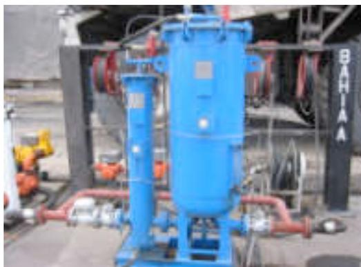
**A typical filter/coalescer/separator in a vertical configuration. Horizontal configurations are also available.**
